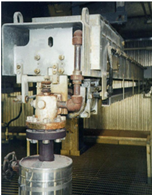
Fig. 5 – Recovery Boiler Sootblower
